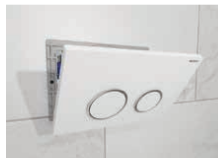
Servicing is easy via flush/access plate.
